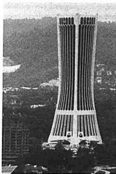
'Deceptively contradictory, a jumble of paradoxes': the Tabang Hajji building in the days when it used to dominate the KL skyline.
